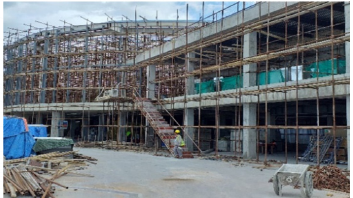
Departures Area Construction in progress
