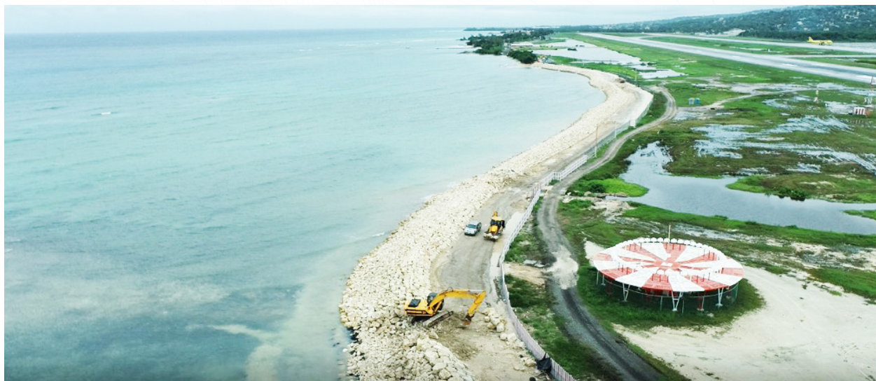
Shoreline Protection Works
