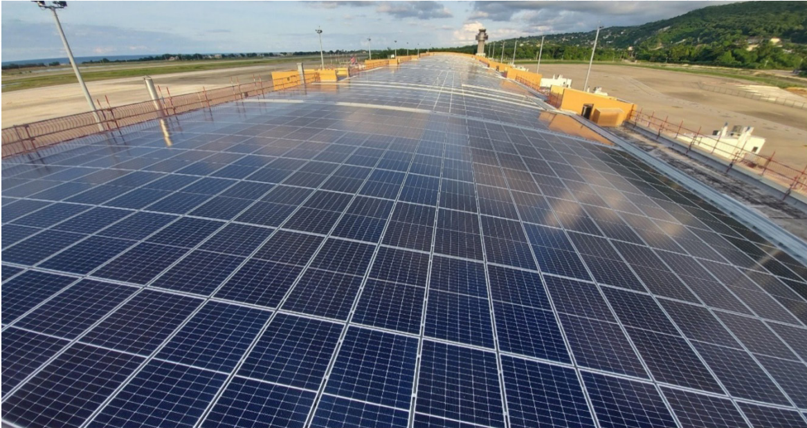
Solar PV Panel installed at MBJ
