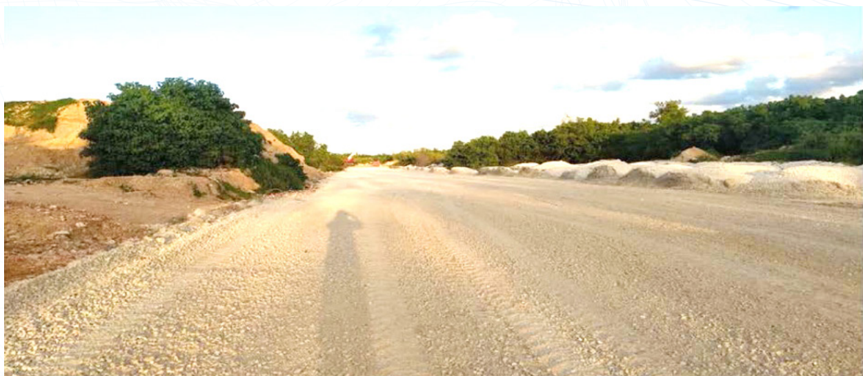
New Road (Kent Avenue) to Whitehouse under Construction
