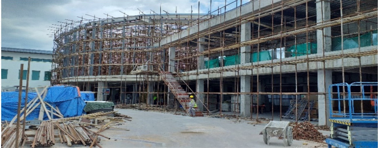
Departures Area Construction in progress
